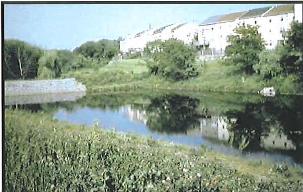
The primary functions of a wet pond are to detain storm water and facilitate pollutant removal through settling and biological uptake
